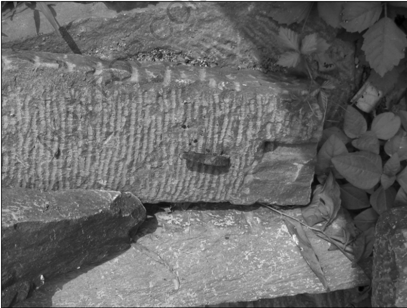
Figure 7. Nails Inserted in the Stone Pillars for Joining Them
