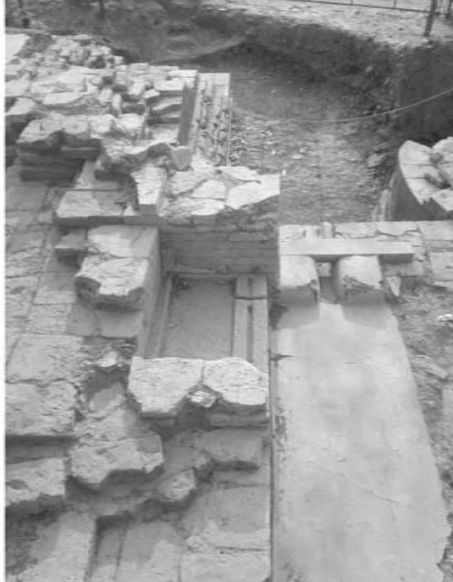
Fig. 15A small three-side closed receptacle (in the middle of photograph), possibly for taking a bath as the rectangular threshold has the longer groove along the sill is meant to receive a door, and the shorter running across to work as the outlet for used water. (after Choudhary and Kumar
