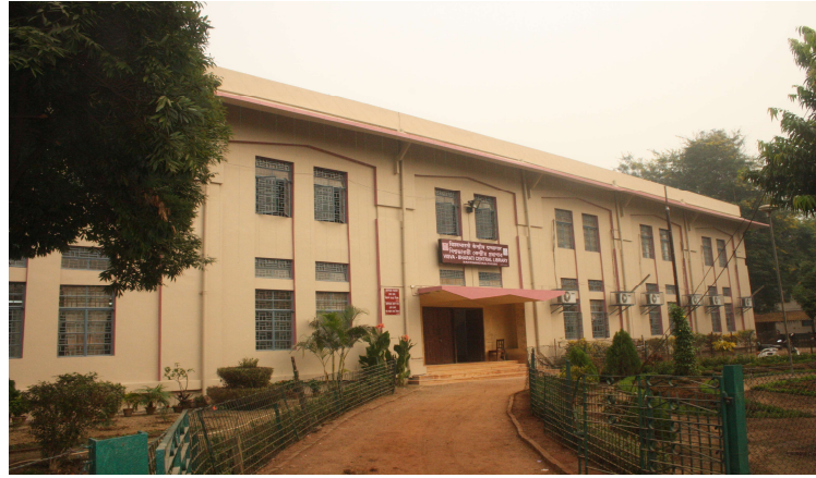
Visva-Bharati Central Library Building after renovation
